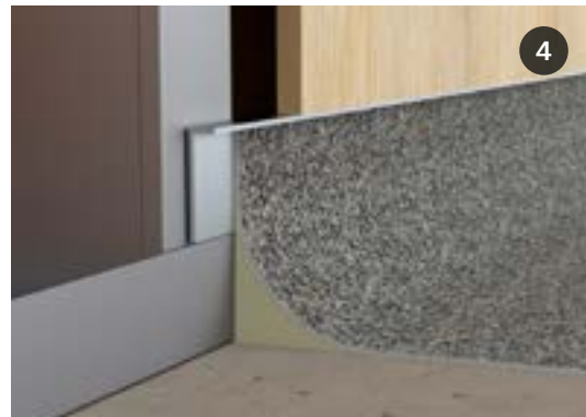
Raised vinyl floor
